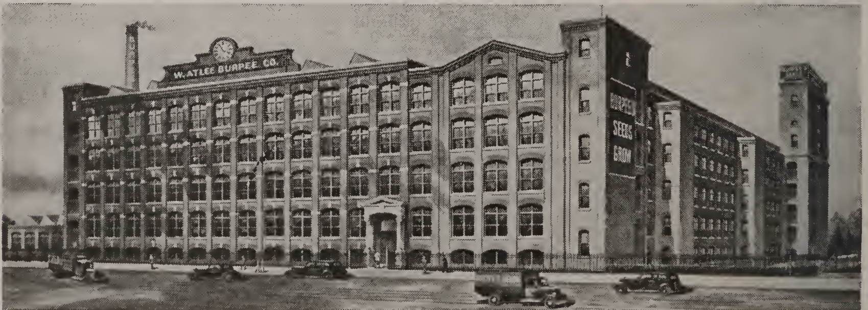
Burpee Buildings, Philadelphia, where all orders for Burpee Seeds and Bulbs are filled.
